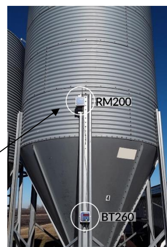
Remote radio placement
